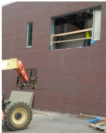
Figure 5: Material being lifted to second floor
